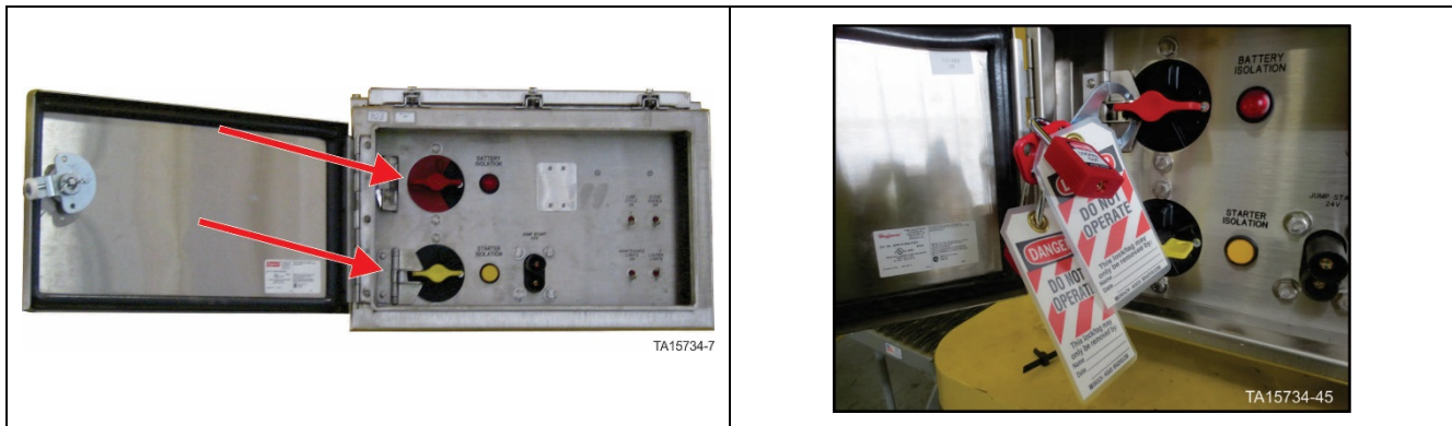
Figure 4. Isolation and control switch assembly
