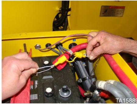
Fire suppression in-line fuse located in loader battery box.
